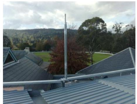
*Forward thinking allowed the Bradman Museum's radio mount to be integrated into the new building design forming part of the structure and saving on the cost of installation.*
